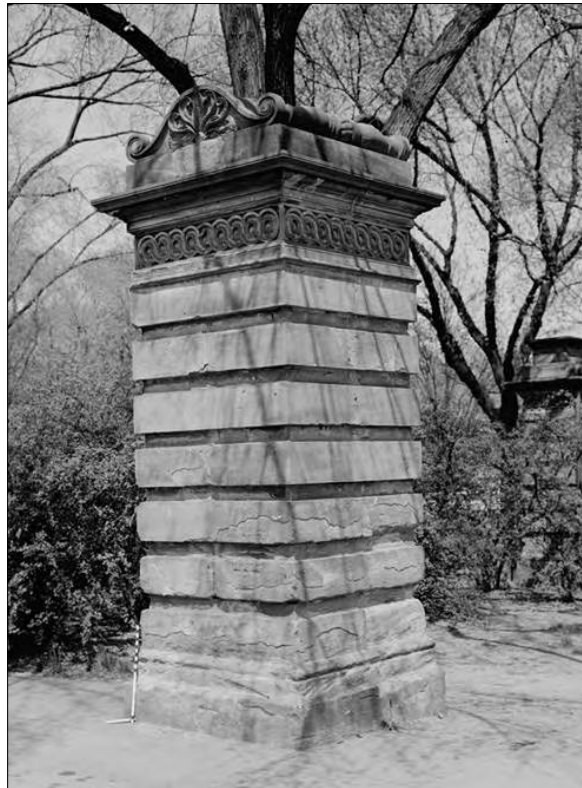
One of the eight remaining Bulfinch gateposts.
